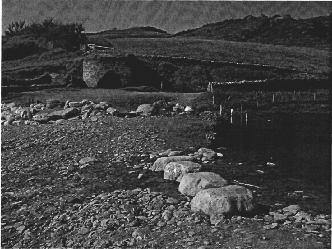
Coast Path prior to breach
